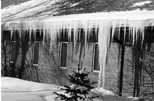
The unusually high heat loss on this roof has caused both an ice dam and icicles.
